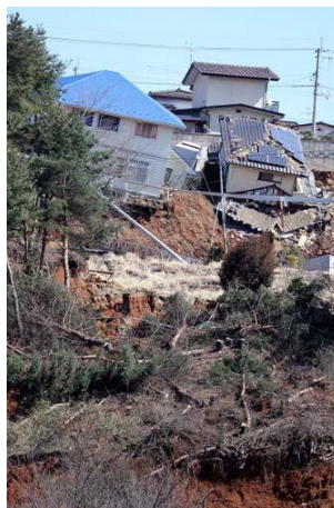
Figure 4.36 Houses are left damaged by landslides in Fukushima, Japan, after an 8.9 magnitude earthquake struck on March 11, 2011, off the coast of north-eastern Japan. The temblor was
