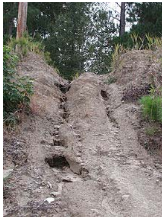
Figure 4.65 Bank erosion started by four wheeler all-terrain vehicles, Yauhanna, South Carolina
