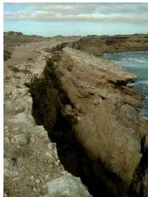
Figure 4.68 Erosion due to wave pounding at Venus Bay, South Australia.
