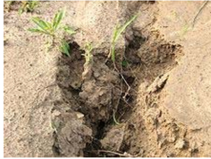
Figure 4.62 Soil erosion exposing roots
