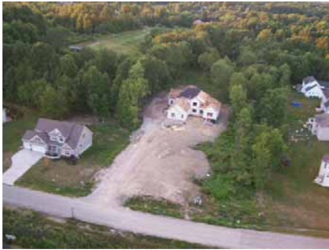
Figure 68: A sample of an aerial view
